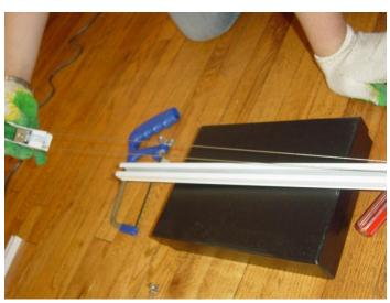
IX) Pull the <u>Steel Wire</u> from the <u>Carrier-A.</u> (again, make sure the <u>Steel Wire</u> is not twisted)
